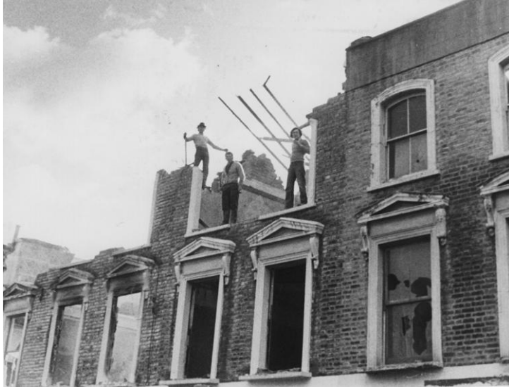
House Demolitions, 1970 (Photo: W.Fawcett)
